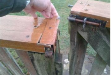
**Finding:** There is sharp sections of plastic on the fence next **Action:** Repair or replace to the gate
