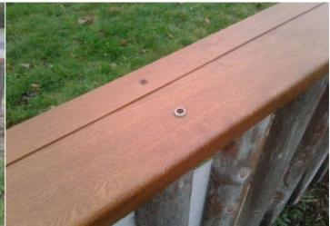
**Finding:** There is/are screw cap covers missing or damaged **Action:** Monitor and replace if required on the item
