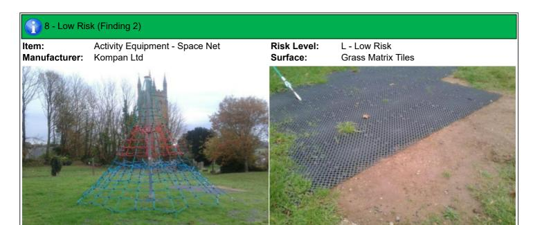
**Finding:** The edges of the grass mat surface have not been **Action:** Tuck in edges of grass mat to remove trip hazards installed in accordance with the API Code of Practice
