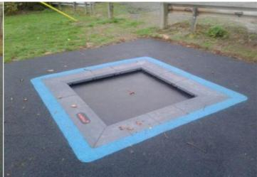
**Finding:** On site visits it is not possible to test the ground clearance of the Bouncing Facility bed as specified in BS EN 1176; ensure that the clearance between the Bouncing Facility Bed and the ground underneath is in accordance with the manufacturers recommendations (it was not possible to measure the depth at time of inspection measured unloaded due to the design of the bed of the bouncing facility).
