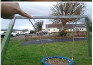
**Finding:** The shackle links are worn in excess of 40% and require renewing ( the shackle is wearing due to the length of the secondary safety chain taking all the weight of the basket instead of the main suspension
