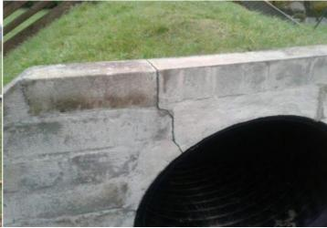
Finding: There are cracks in the wall
