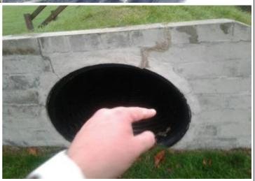
**Finding:** There are some rough edges of the plastic and concrete at the entrance on the tunnel
