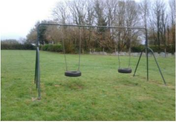
Finding: The surface has eroded and the foundations are exposed
